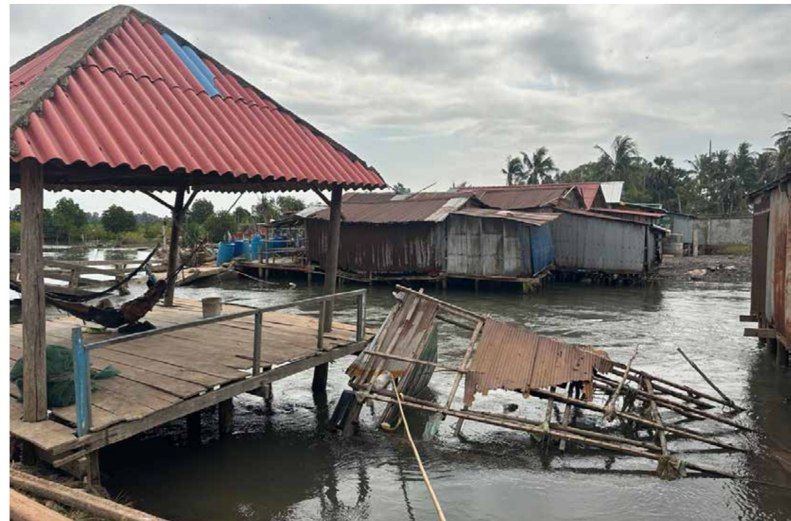
Picture 27 - Communities in Angkal face financial precarity and inadequate housing infrastructure
