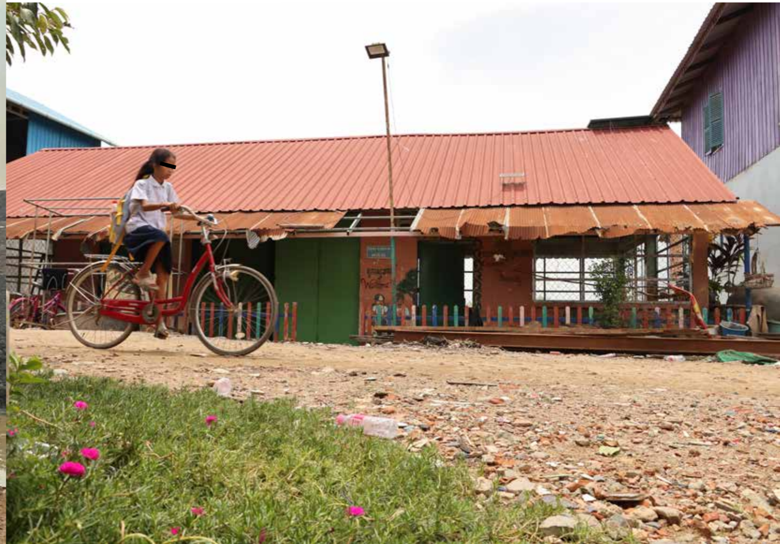
Picture 20 - School in Canal 94 is derelict, June 2024
