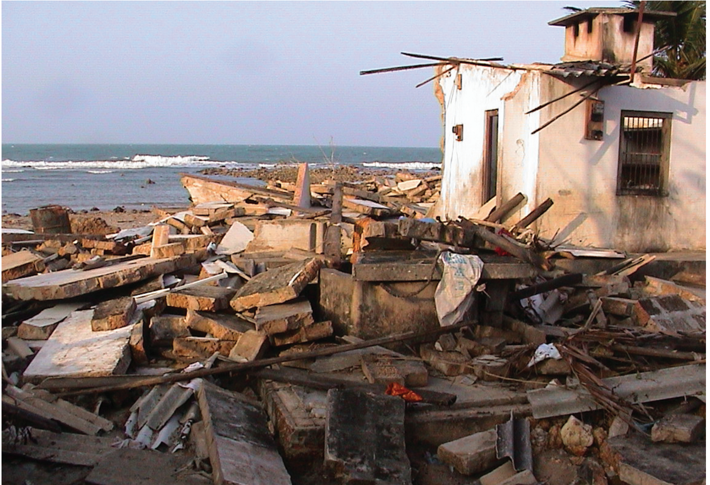
A beach house at VVT.
