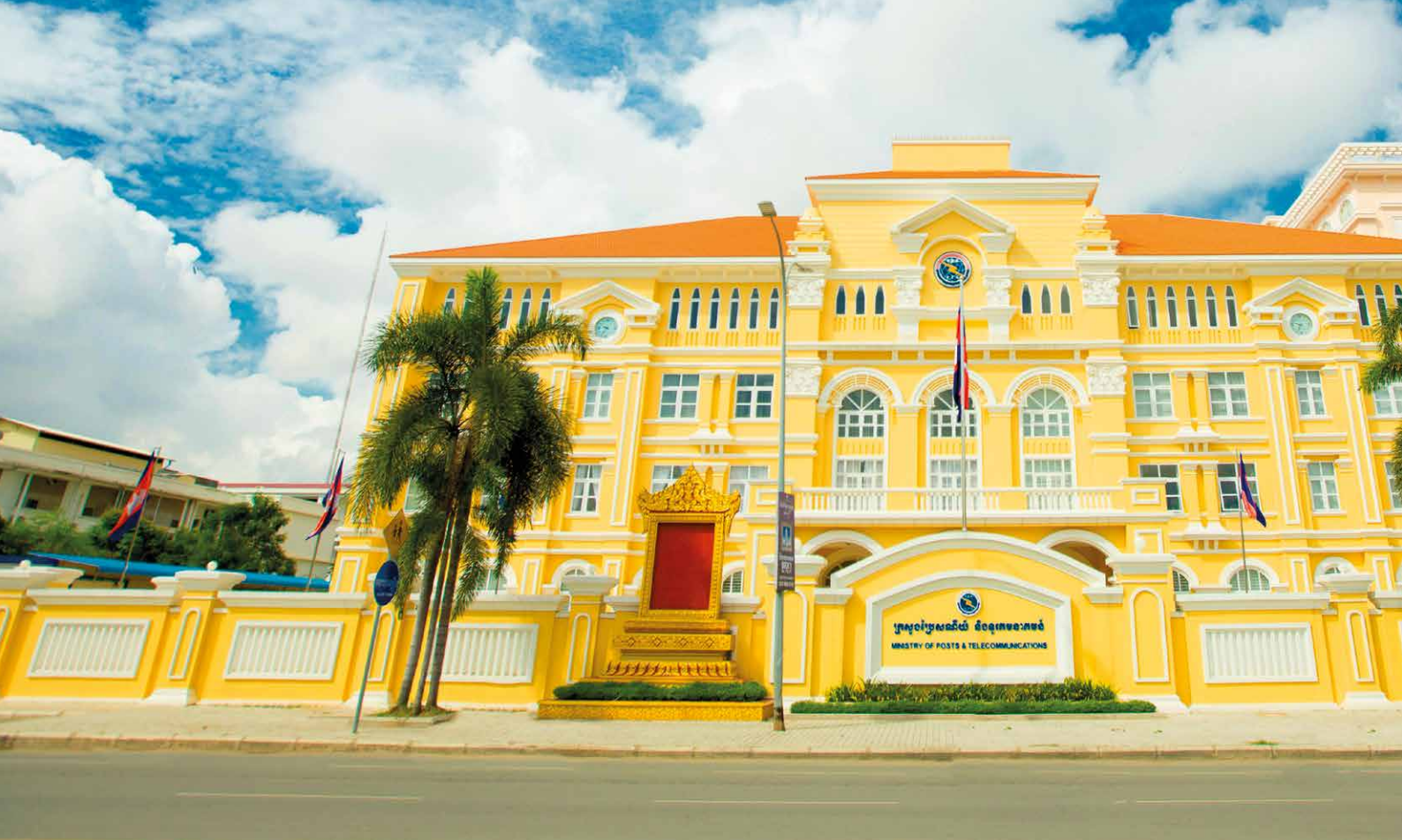
The Ministry of Post and Telecommunications in Phnom Penh (Photo: Chetra Chann on Unsplash).
