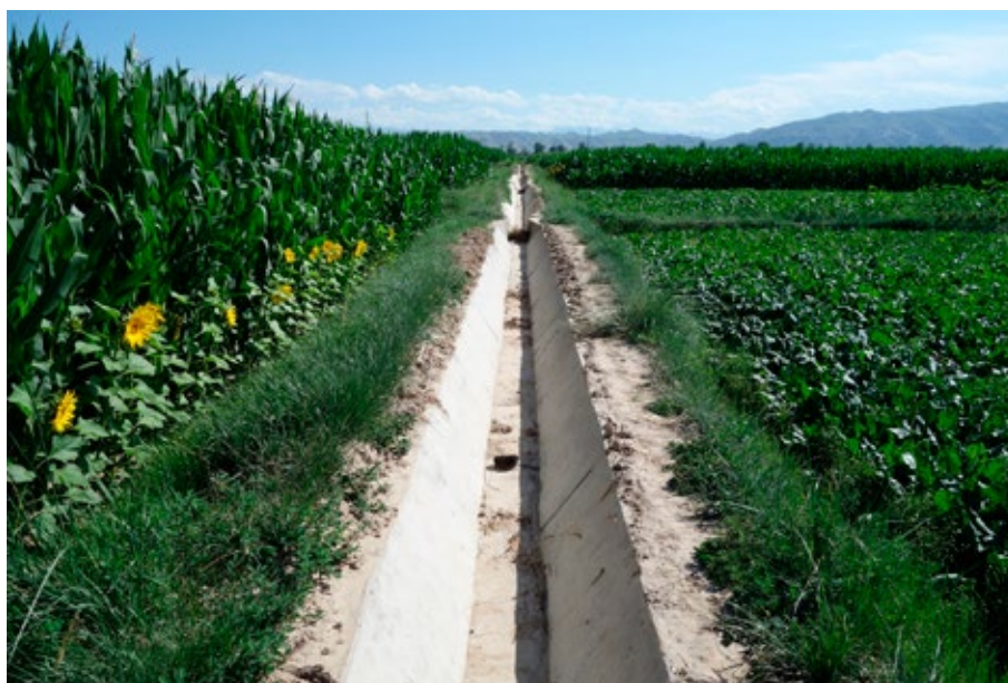
Modernized irrigation canal
