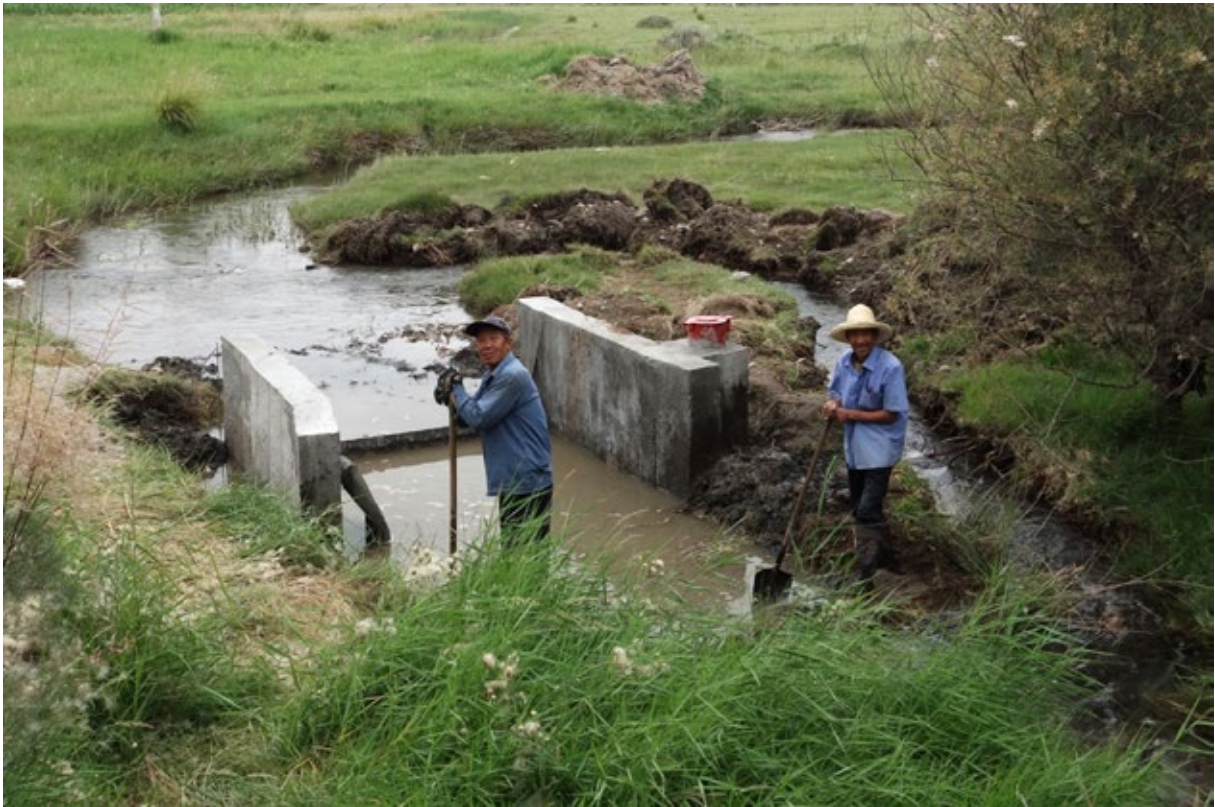
Adjusting the irrigation canal
