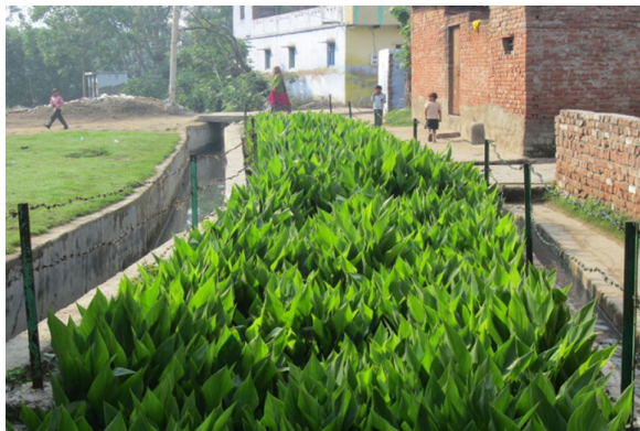
Figure 10.8 Primary treatment unit (baffled septic tank).
