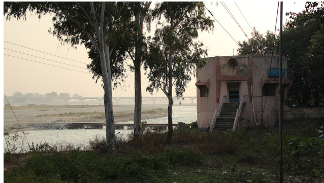
Figure 16.3 Example of a large diameter caisson well adjacent to Ganga River (Photo: HTWD, 2011).
