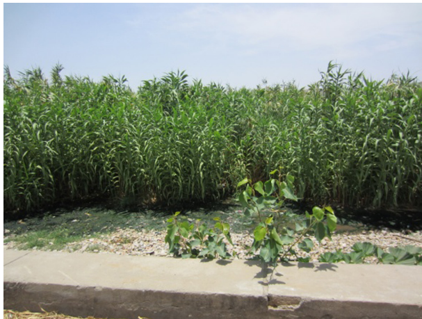
Figure 10.4 HSSF-CW (second step in tertiary treatment).
