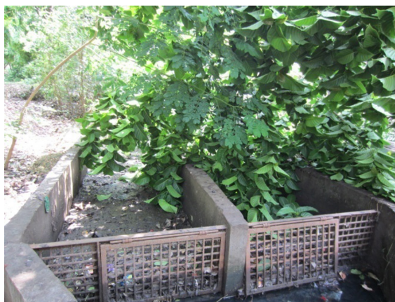
Figure 8.6 Poor maintenance of the primary treatment unit prior to HSSF-CW in Ekant Park, City of Bhopal, central India.
