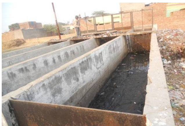
Figure 8.12 Poor maintenance of the primary treatment unit prior to WSP in the Municipal WWTP in City of Agra.
