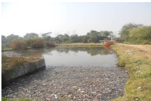
Figure 8.11 Poor maintenance of primary treatment unit lead to carry-forward of garbage and solids in WSP in the Municipal WWTP of the City of Vrindavan.
