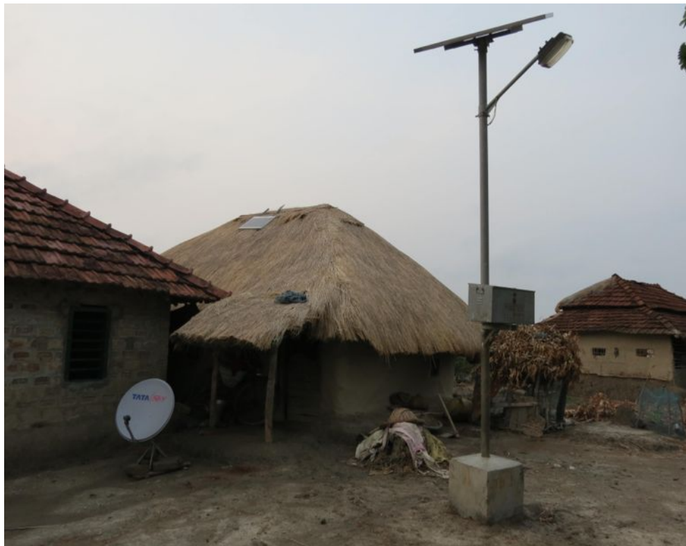
Figure 12: The solar home-lighting system, installed to help families work, is used chiefly for watching television. Note the solar panel on the thatched roof and the dish antenna on the ground, next to the solar streetlight
