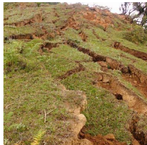
Figure 3: Cracked land (Source: DADO Gorkha)
