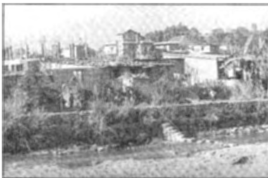
Typical Settlement along Riverside
