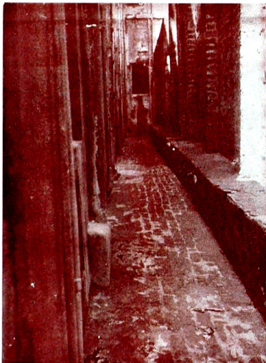
The Scene of Murder The Sewered ditch showing the aperture and blood Patches
