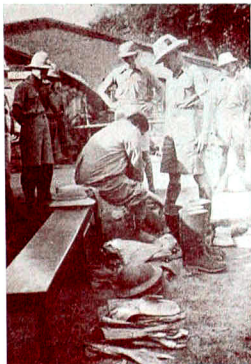
Sub Inspector J. B. Dutta wearing protective attire A.R.P. training, Calcutta Police
