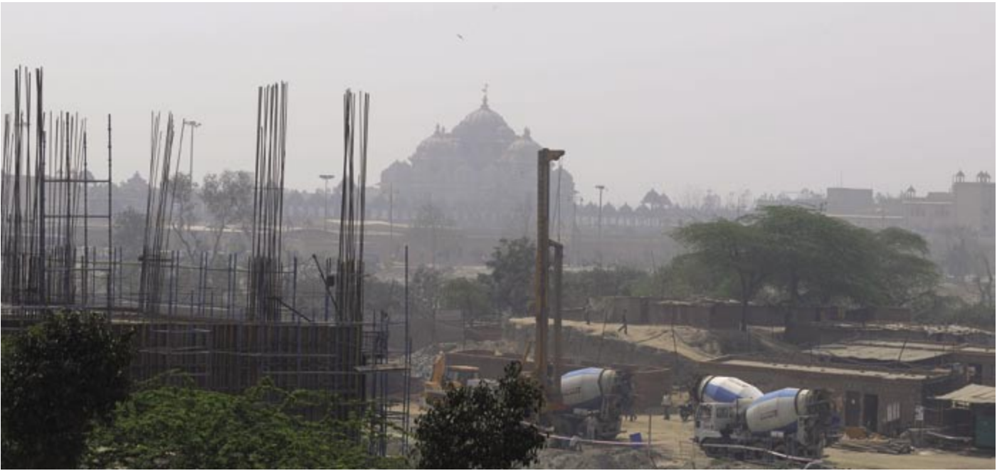
Construction site of the Commonwealth Games village with Akshardham complex in the background.
